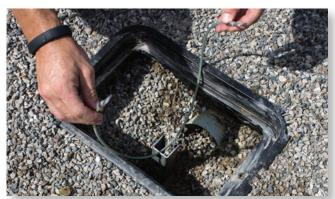
**Step 2:** Loop security cable through one of the loops in the galvanized stake.
